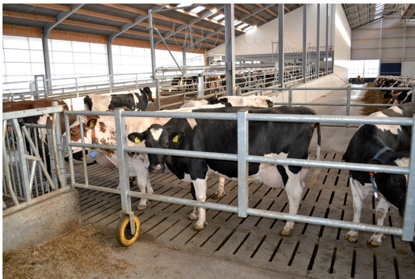
• Passage way in a feed alley using 2 telescopic partition barriers
