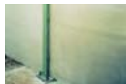
2. Slotted in between.
