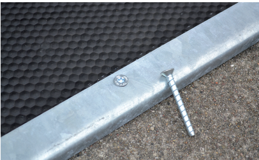
• Galvanized fastening profiles are installed with concrete screws
